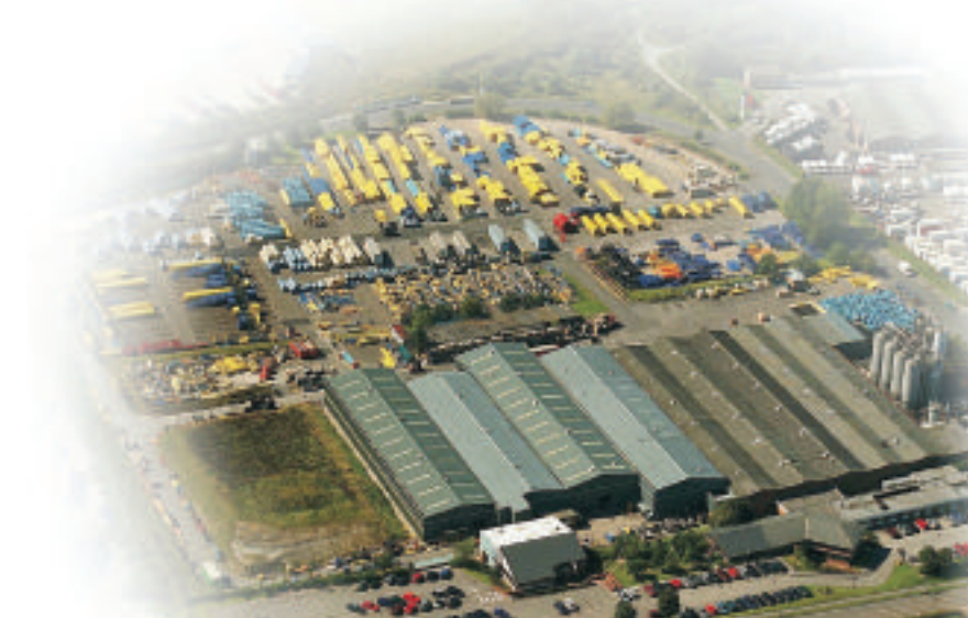
▲ The manufacturing facility at Hilcote, Derbyshire, is one of four plants included in the deal
