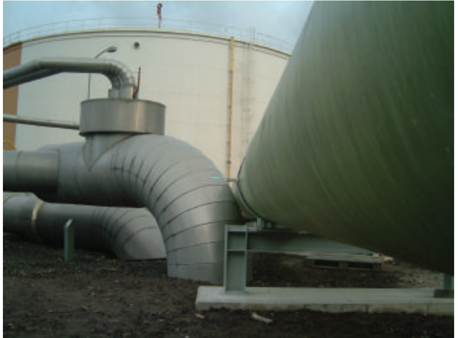
▲ Flexible assembly: FRP flue gas pipeline
