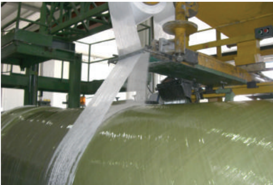
▼ Large span between supports: FRP pipe with diameter 1,400mm
