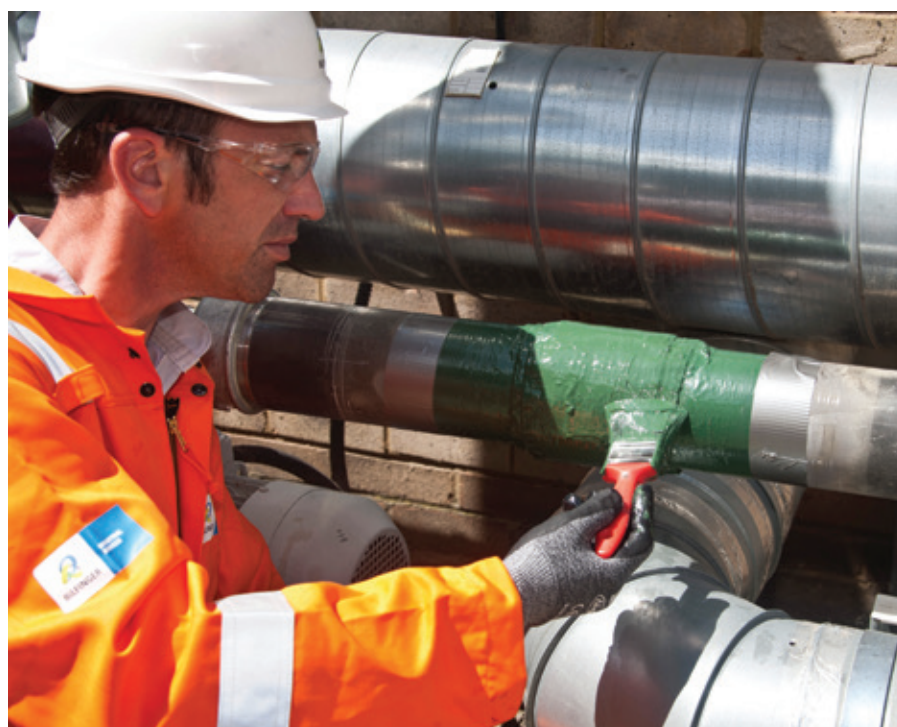
Applying the Loctite Composite Pipe Repair System
