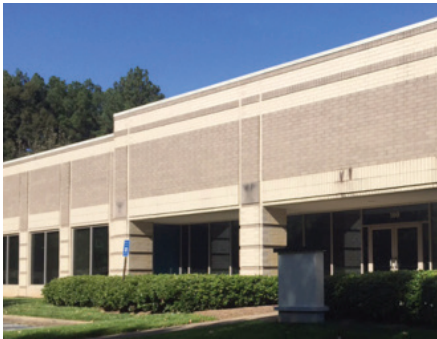
Office & Warehouse Dock Loading Franklin Oaks 889 Franklin Road, Marietta, GA 26,588 Square Feet
