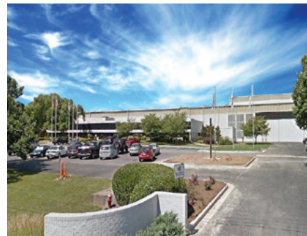
Manufacturing Plant 501 Richardson Road SE, Calhoun, GA 284,349 Square Feet on 80 Acres
