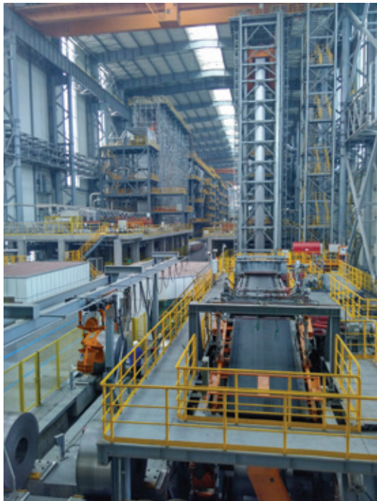
The existing galvanising line supplied by Primetals Technologies in the cold rolling mill of Tangshan Iron and Steel Group
