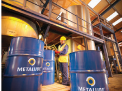
○ One of the new blending tanks at the site
