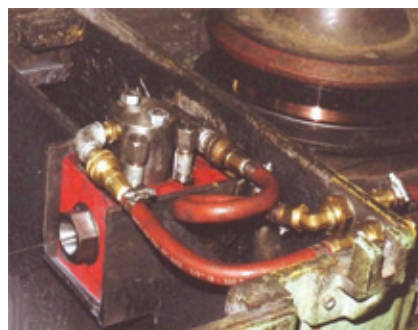
○ Wire cleaning by PWC-S system
