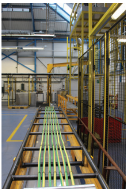
○ The ladder rack being prepared before the test
