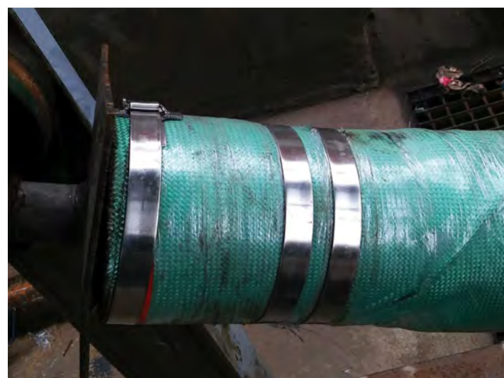
Copper Cable Connectors use Band-It products for water cooled furnace cables.
