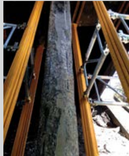
A column of the Ashburton Bridge on the N3 pictured after a blazing truck had caused extensive fire damage last year, and in its new repaired state after the use of three a.b.e. Construction Chemicals concrete repair products.
