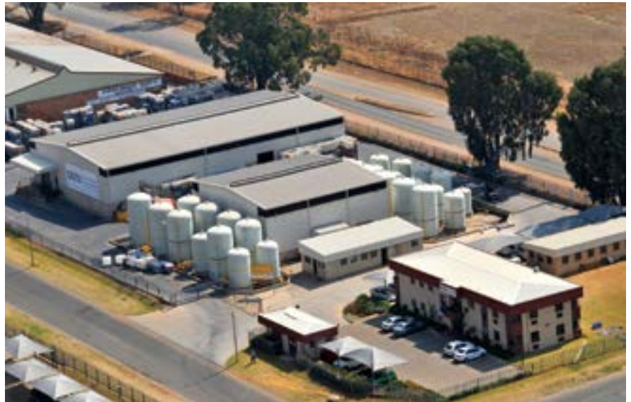
Chryso Southern Africa's operation in Jet Park, Johannesburg.
