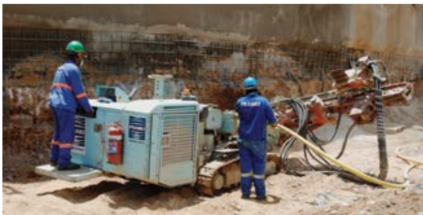
Drilling for the installation of the strand anchors. In instances, 25 m long anchors were installed.
