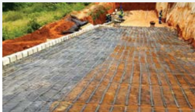
The Tensar polyethylene RE560 uniaxial geogrid.
