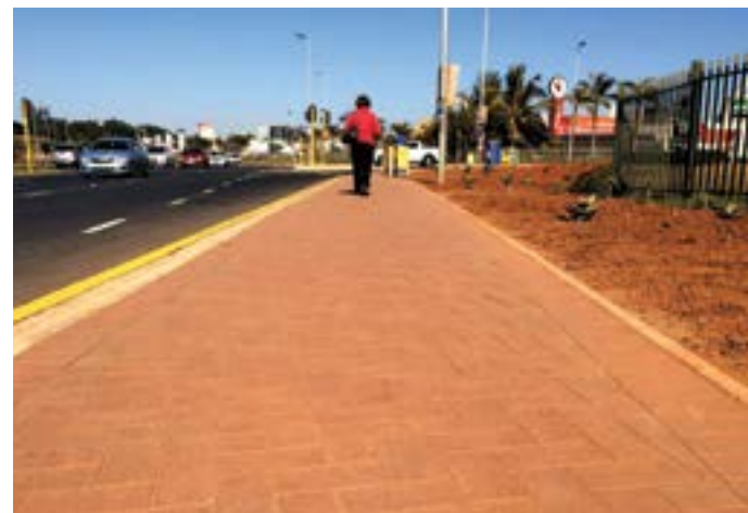
Corobrik's Burgundy pavers have been used to construct the sidewalks and islands along both sides of Ballito Drive, extending from Greenfields Road near the new N2 interchange, all the way to the M4 intersection.
