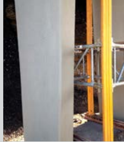
A column of the Ashburton Bridge on the N3 pictured after a blazing truck had caused extensive fire damage last year, and in its new repaired state after the use of three a.b.e. Construction Chemicals concrete repair products.
