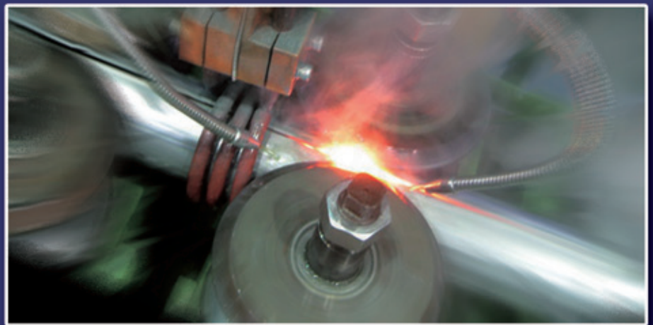
Automatic Stainless Pipe Welding Scene
