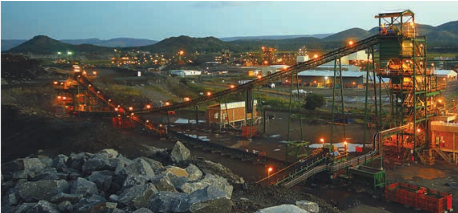
Night view of the Tharisa mine, which is located on the south-western limb of the Bushveld Complex, near Marikana (photo: Tharisa).
