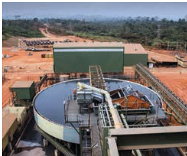
The Asanko processing plant showing the pre-leach thickener. Steady-state operations at Asanko are expected by the end of Q2 2016 (photo: Asanko Gold).
