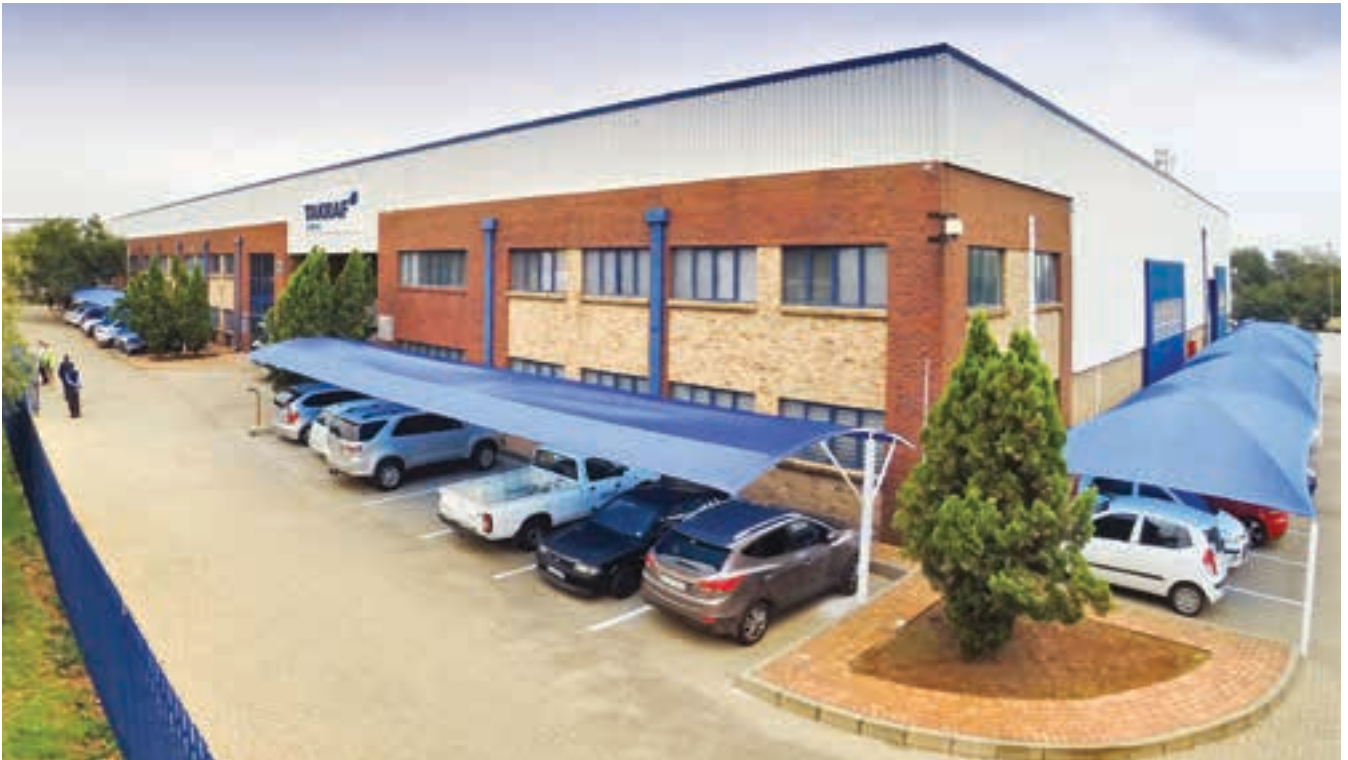
Tenova TAKRAF Africa has consolidated operations in these modern premises in Spartan.
