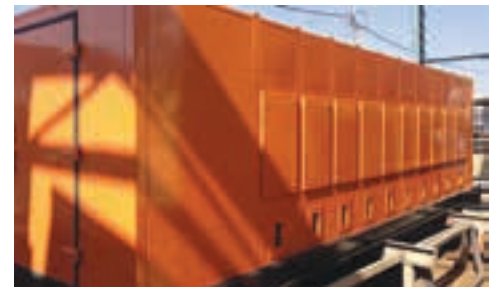
Designed by Shaw Controls for underground application in a coal mine, the E-House was designed with several specific parameters taking precedence.
