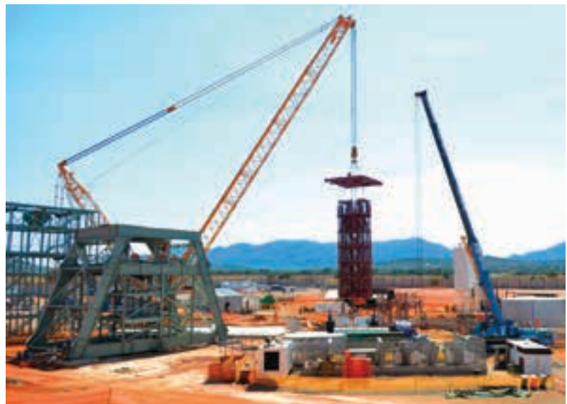
The stage and bank steel being lowered into Shaft 1.
