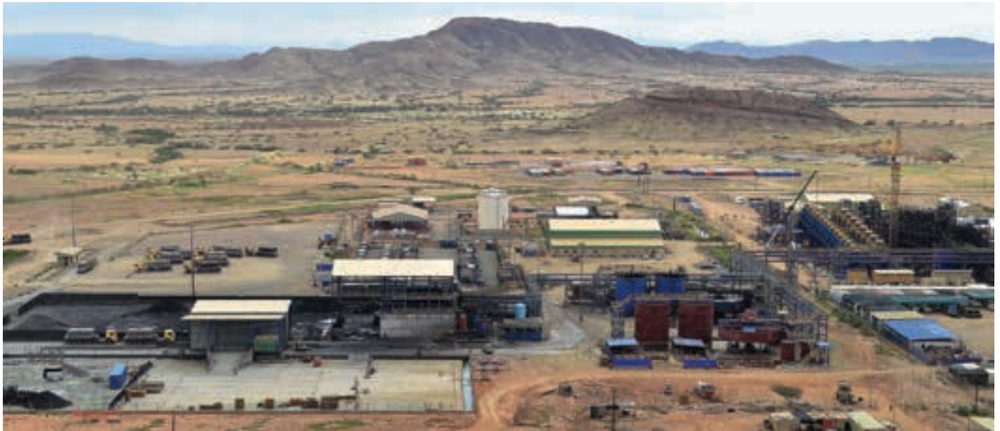
Overall view of the zinc expansion project at Bisha (photo: Nevsun).
