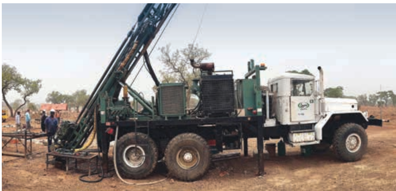
A drill rig in action during a recent drill programme at Kobada for metallurgical and geotechnical testwork.
