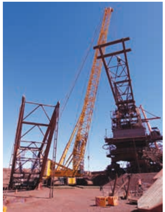
Placement of the old counterweight boom structure.
