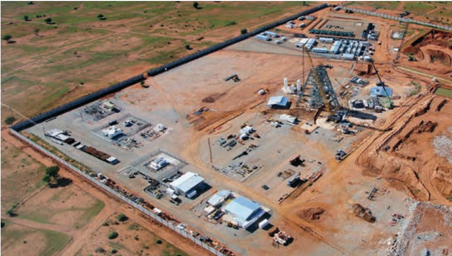
Aerial view of the Platreef site. It has been entirely fenced with an inner concrete wall surrounding the shaft area.
