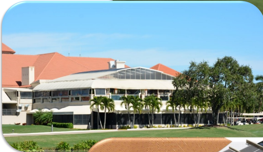
PHOTOGRAPH OF EXISTING STRUCTURE
