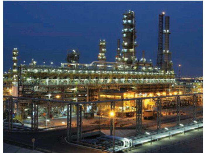
○ The Laffan Refinery in Qatar. Photograph courtesy of www.2b1consulting.com
