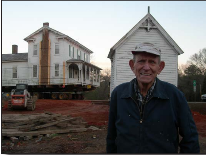
Billy Hartness in front of his former home, the historic Pugh house built in 1870, being moved to a new location. Needed road improvements threatened the structure, so Town staff worked with Mr. Hartness to find another location.
