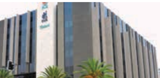
The @Parkside building in Freedom Square, Windhoek, is the first building in Namibia to achieve a Green Star rating, having been awarded its 4-Star Green Star Office SA-Namibia 'Design Rating' from the Green Building Council of South Africa.
