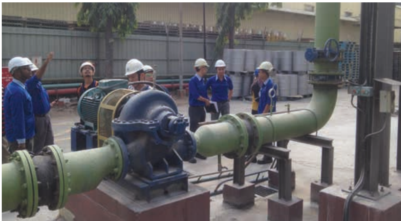
Following theoretical training on pump operation, pump and system interaction and the benefits of improved efficiency, delegates walk through the plant looking for visible signs of energy wastage, such as throttling control valves, overflows, recirculation, etc.
