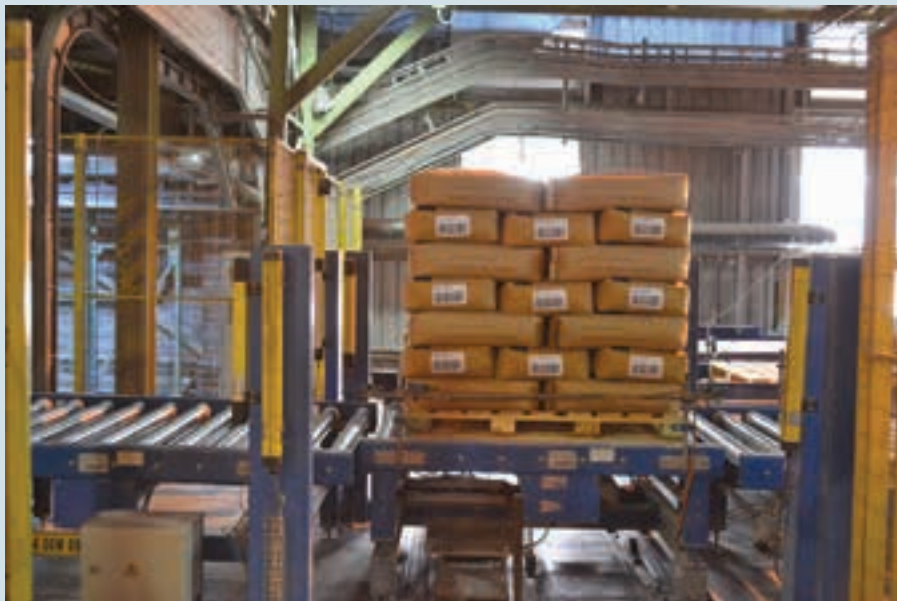
When a pallet of a particular wax is fully loaded, it is rolled onto the transfer trolley. The transfer trolley then moves the pallet across to align with the exit conveyor.
