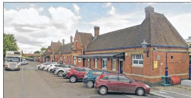
The main entrance to Newbury station is looking a 'little tired'
