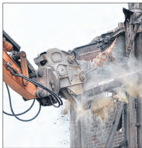
Demolition work has started on the Sterling Cables tower
