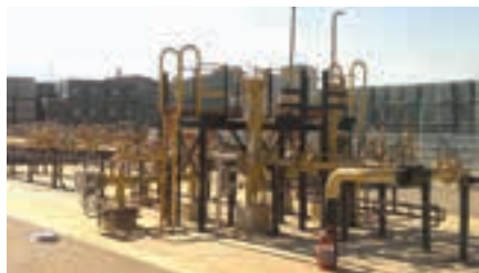
The newly constructed Nampak pressure reduction station (PRS) in Germiston.
