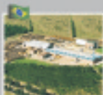
MADEM SA BRASIL | Itapetininga, RS 1000 000 plywood reels/year 130 000 wood reels/year
