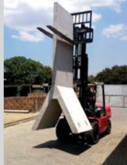
The YFEL wall units are transported on site and put in place using a forklift truck or crane.
