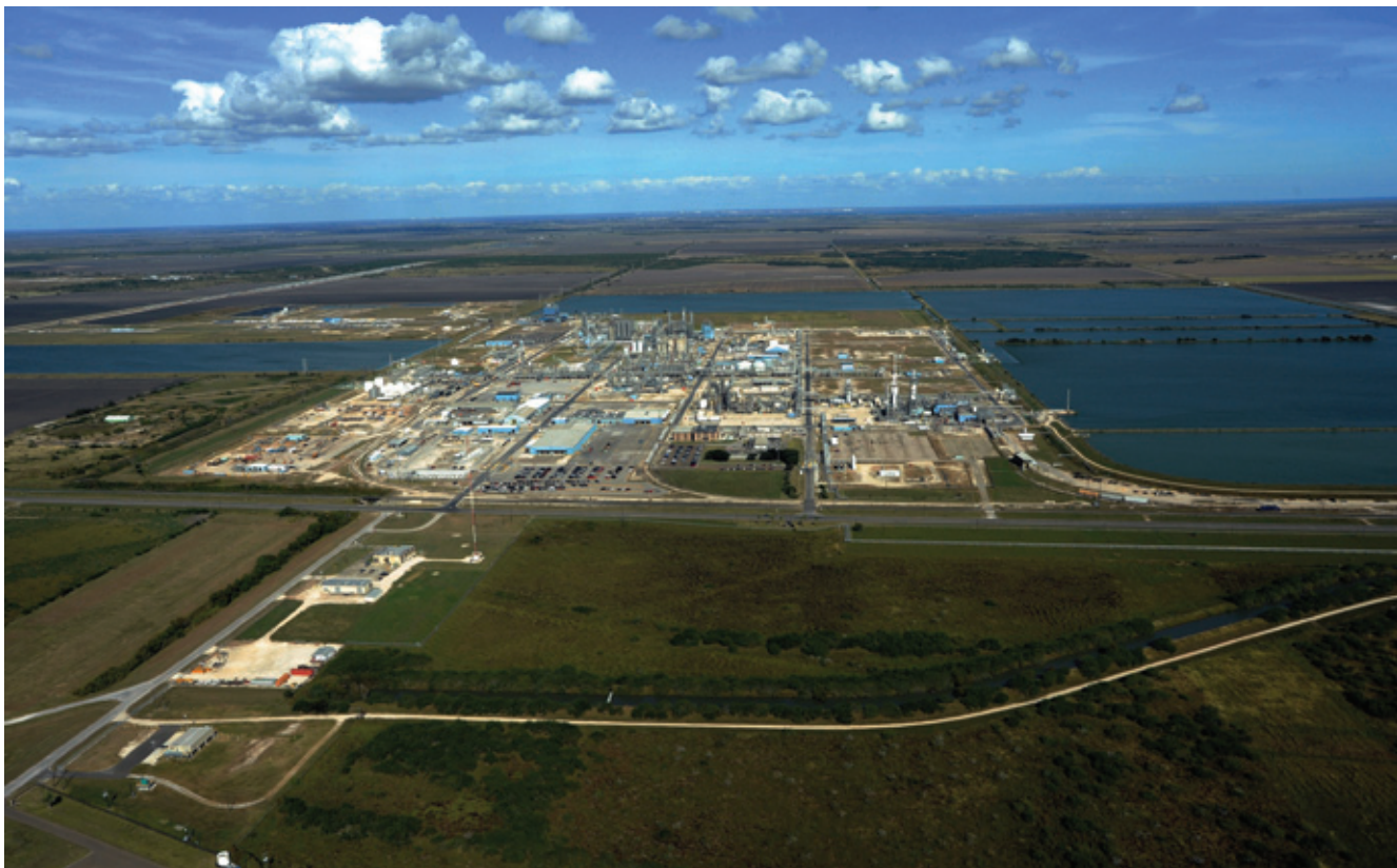
▲ The Seadrift, Texas, site of Dow Electrical and Telecommunications
