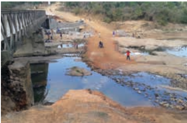
Bridges that needed to be crossed had been washed away and roads were impassable, complicating the delivery of Kwikspace's units to site.
