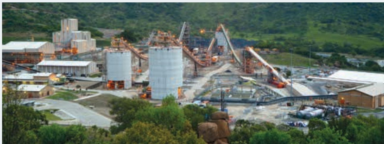
The concentrator plant has a nameplate capacity of 187 500 tonnes per month.
