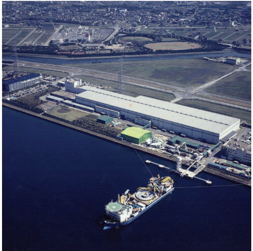
▲ The new Nexans plant at Tokyo Bay
