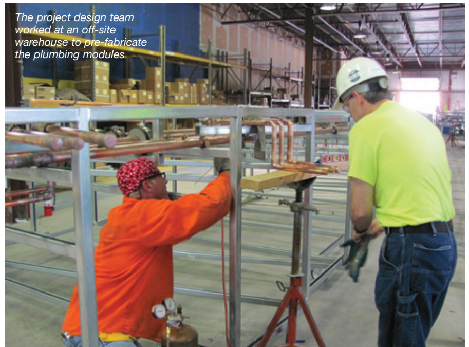
Copper tubes were installed for domestic hot and cold water service, HVAC systems and medical gas distribution
