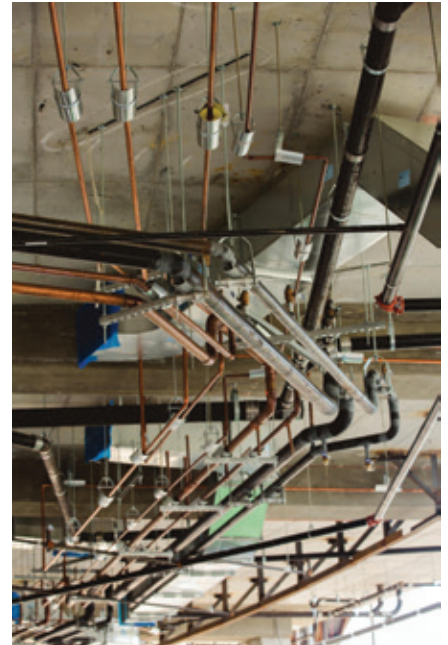
Copper tubes were installed for domestic hot and cold water service, HVAC systems and medical gas distribution
