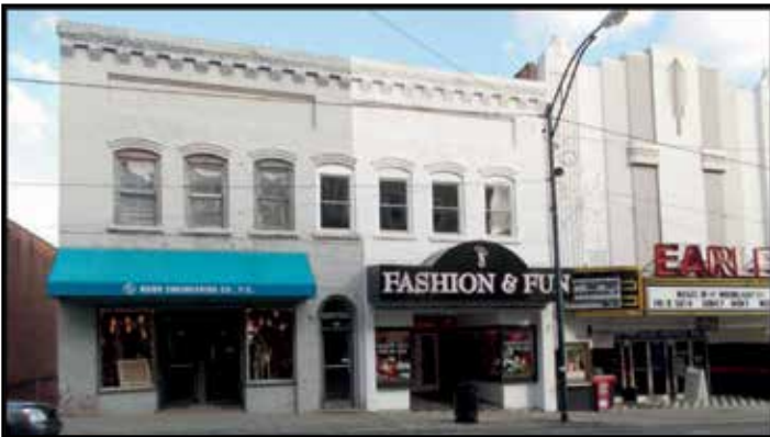
COMMERCIAL BUILDING AT 148 N. MAIN ST., MT. AIRY; 2 story approximately 2500+ SF . Downstairs long term tenant, upstairs rented by building next door for storage. Shared stairs and hallway with building to left. Price is based on 8% cap rate of gross income. Offered at $142,500 . Great location near all the downtown action and Snappy lunch! Call Debbie at 789-1365 for showing of more info.
