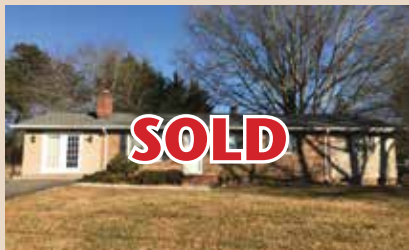
871205 167 TERRI LN., MT. AIRY - Beautiful 3 BR, 2 BA home in quiet neighborhood close to town but not in city limits. Master BR & another BR have been expanded, both BA's remodeled. Appliances stay. New HP w/propane backup. Gas log FP in LR. Enclosed carport is being used as a DR w/French doors. Storage bldg stays, back yard is fenced..... $135,900
