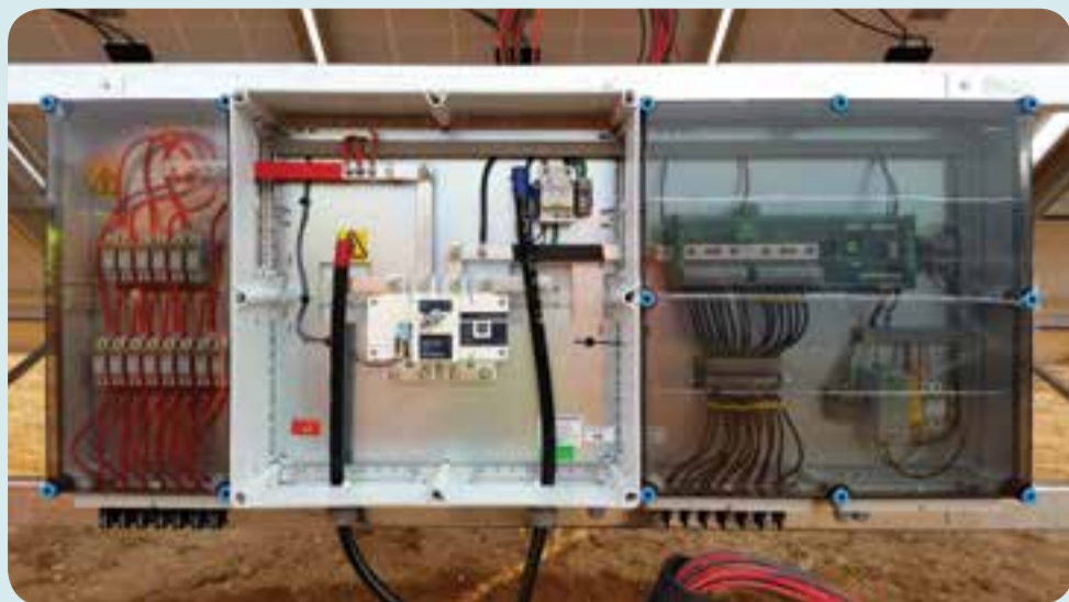
A string combiner box, produced at the state-of-the-art assembly plant at HellermannTyton's premises in Johannesburg, which is destined for a 90 MW solar farm currently close to completion in De Aar.
