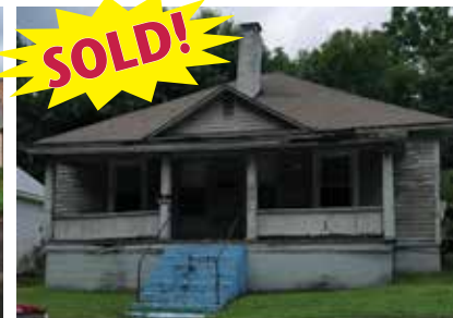
359 E. Oak St- Handyman Special! - 2 Bedrooms, 1 Bath, Large Living Room w/ Hardwood Floors, Large Kitchen, Laundry Room, Covered Back Porch, Covered Front Porch. Oil Monitor Heat and Window Air; New Thermal Windows, some new plumbing! Priced to sell at only.....$19,900
