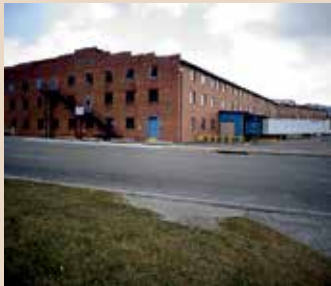
100 T. GEORGE VAUGHAN JR. RD., GALAX, VA - 408,276 sq. ft. industrial building. 3 stories, 12 dock doors, 2 drive-in doors. 5.2 acres. Conveniently located near downtown Galax..... $999,000
