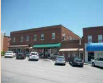
761376 N. MAIN ST., STUART, VA. Apartment & commercial store front. (5) 1 BR, (8) 2 BR's, 3 efficiency apartments recently remodeled. 8 commercial spaces. Call for rental information..... $550,000
