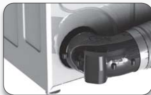
Installed on Dryer
