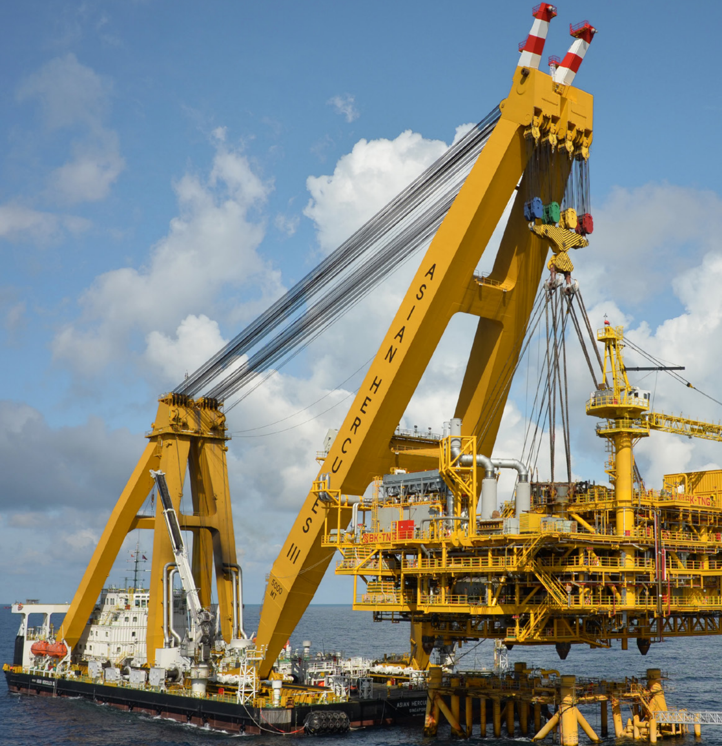
Installation of the 4,200 ton Thien Ung platform topside by the sheerleg crane Asian Hercules III offshore Vietnam.
