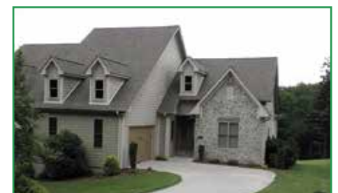
133 Wimbledon Drive - High end finishes abound throughout to include large crown moldings, granite counter tops, 10ft. ceilings, vaulted ceilings, stone fireplace, 8ft. doors, and over sized millwork. This beautiful 3 bedroom/3 bath townhome overlooks the 3rd Green with views of Holes #2 Green & Pond plus the #4 Fairway, and the mountains. Relax & enjoy sunsets from the large deck as the lawn maintenance is covered by HOA ..... $299,000
