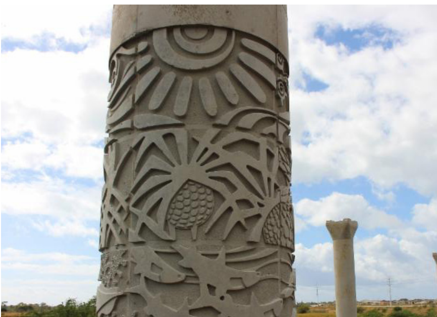
HRTP's embossed guideway columns near future stations Image courtesy of HART
