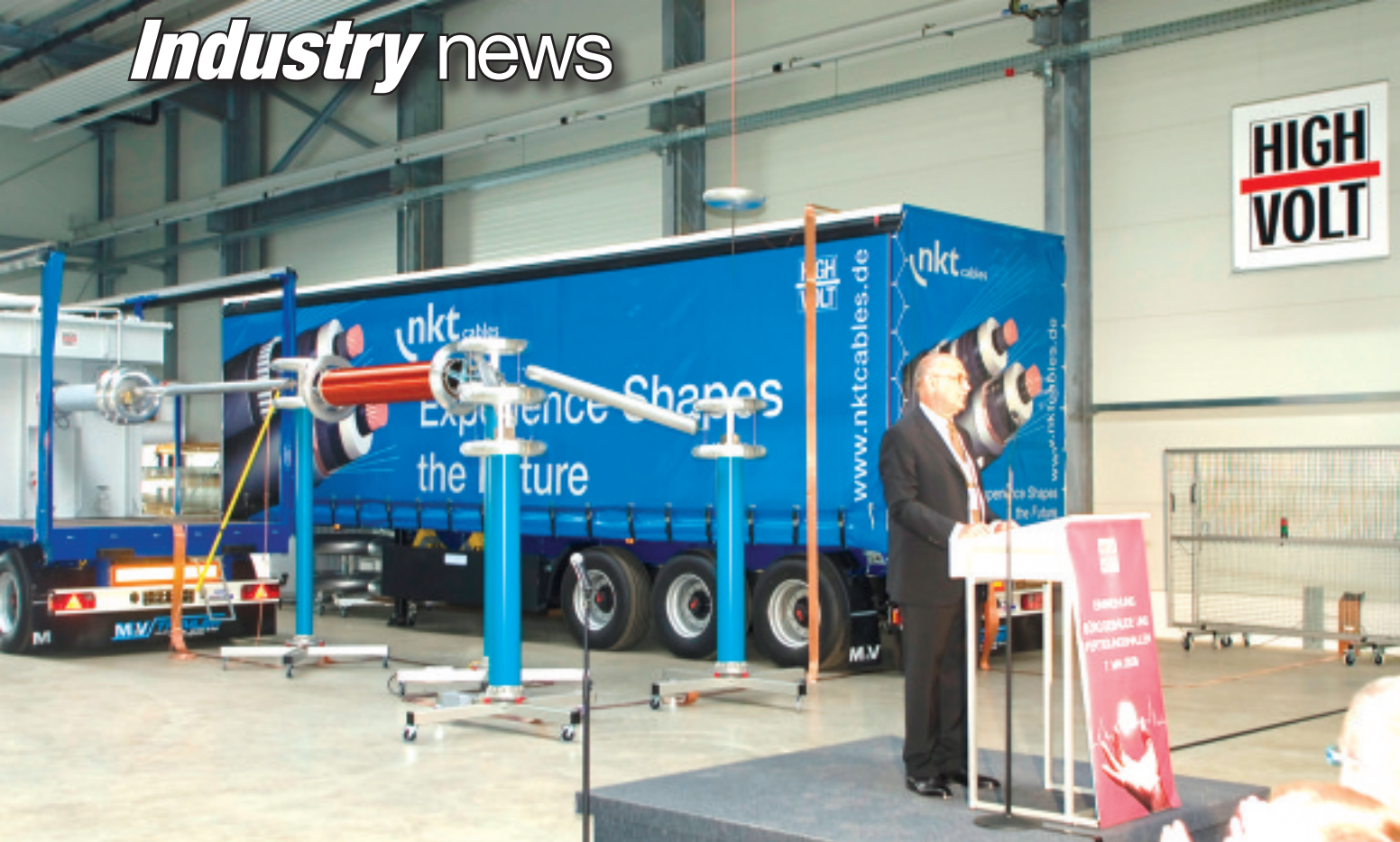
○ Frequency controlled HV AC resonant test system, being demonstrated by general manager Dr Bernd Kübler at the inauguration ceremony
