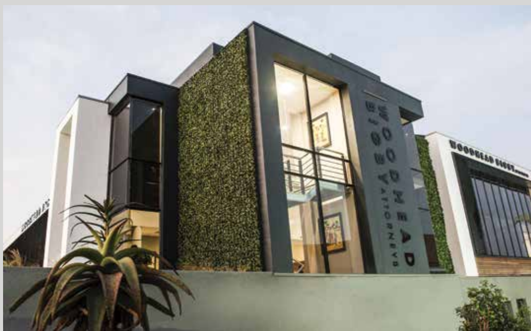
Magnet recently completed the design and installation of an energy efficient lighting solution at the new offices of Woodhead Bigby Attorneys in Umhlanga, KwaZulu-Natal.
