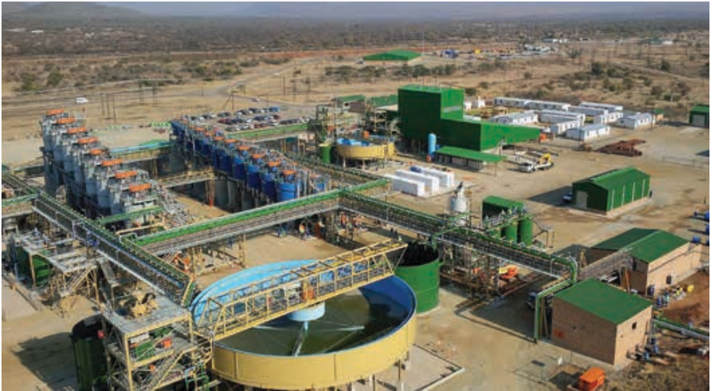
The processing plant at the Maseve mine utilises a standard MF2 circuit configuration and is designed to treat ore at a rate of 165 000 tonnes/month. This photo shows the flotation circuit, concentrator and filter press (photo: Platinum Group Metals).
