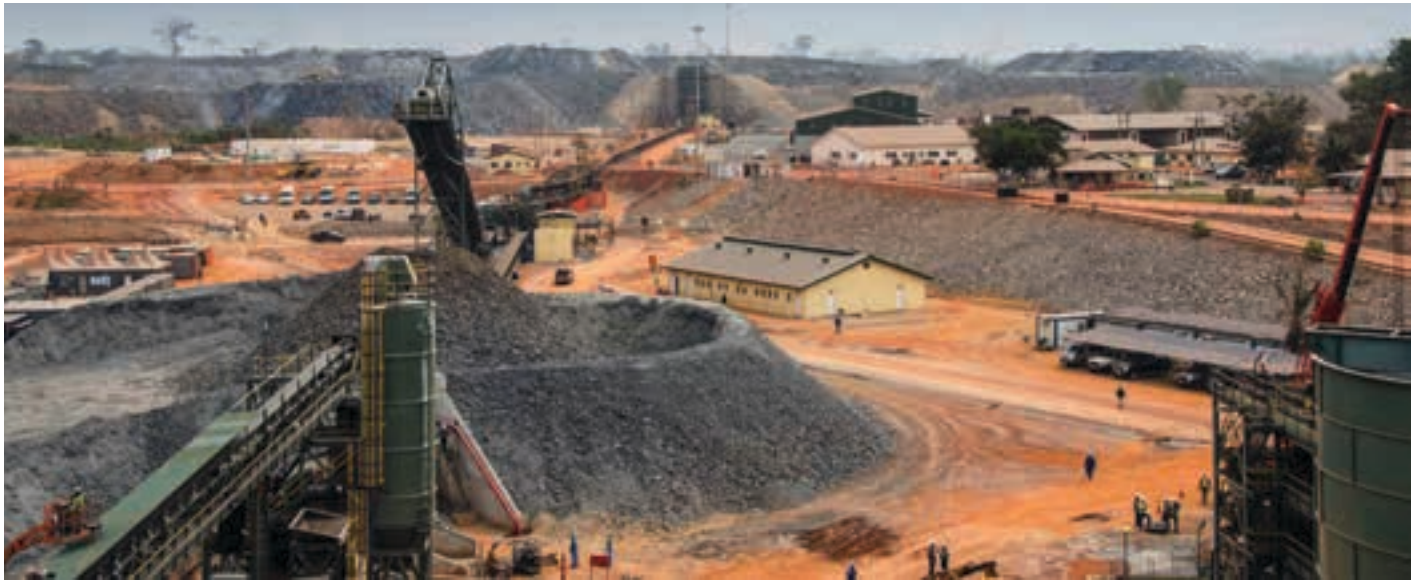
The Asanko Gold Mine showing the ROM pad, crusher and conveyor of the Phase 1 processing facility (Photo: Asanko Gold).
