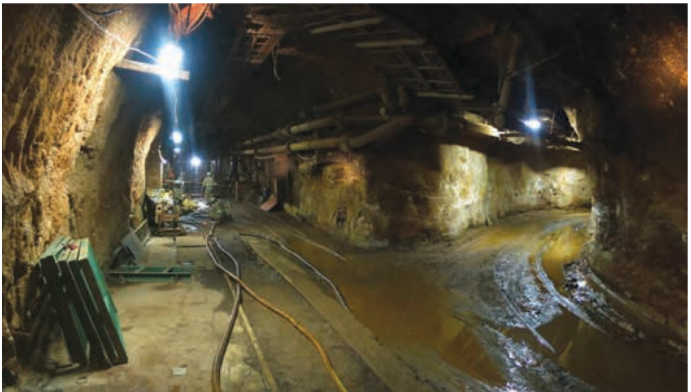
Underground at Kipushi showing Y-junction on 1 200-m level. Silos to the right and cage to the left (photo: Ivanhoe Mines).
