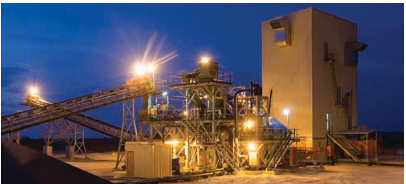
The processing facility of the Ghaghoo underground mine showing the sort house (photo: Gem Diamonds).
