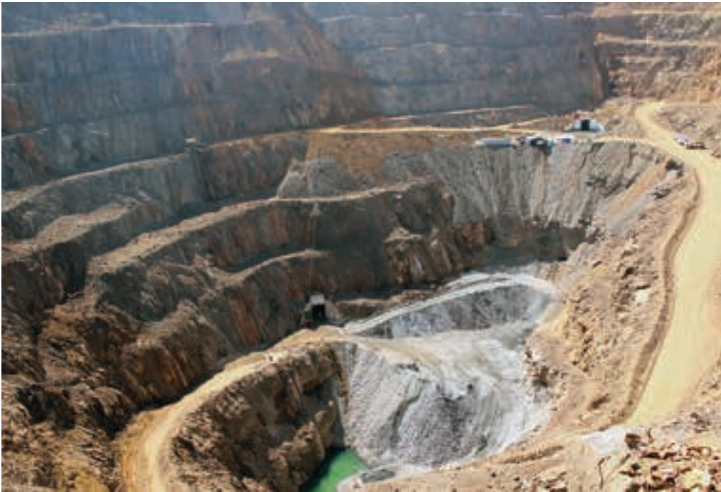
Above: The Tau pit at the Mupane gold mine near Francistown showing the portal to the underground mine (photo: Galane Gold).
