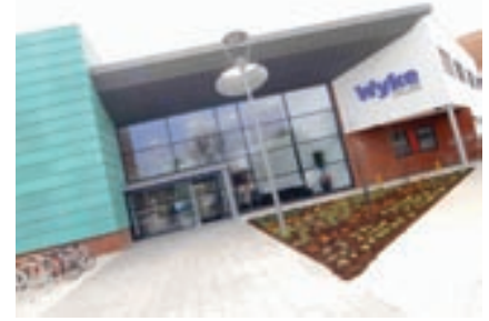
Wyke College has installed a ground source heat pump system
