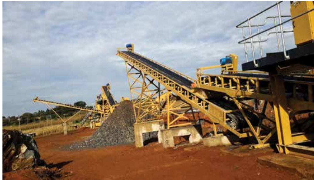
A 250 tph modular Trio aggregate plant installation in East Africa.
