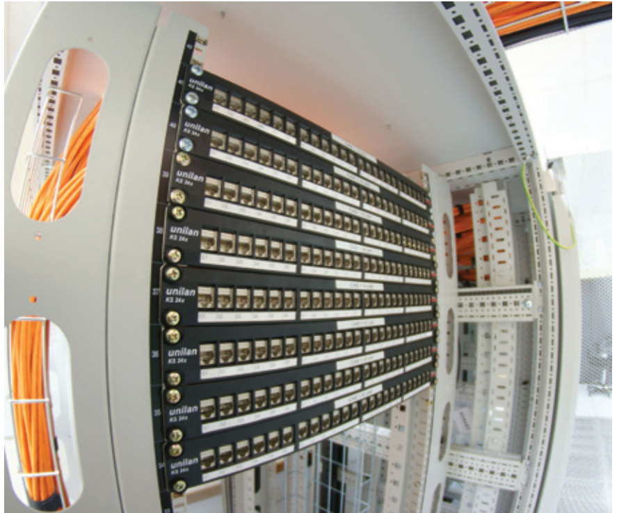
▲ Some of the installation from Dätwyler
