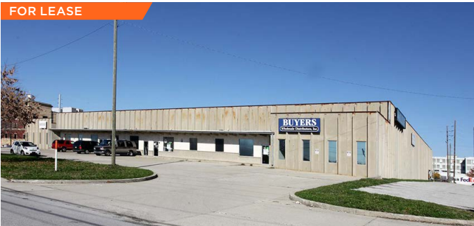
510 W. Merrill Street 23,800 SF Indianapolis, IN
