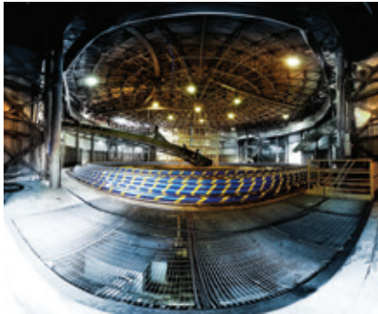
○ The cable being laid across the Messina straits
