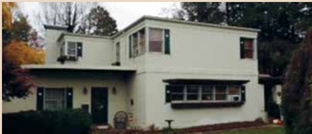
695728 339 COUNTRY CLUB ROAD - One of the more famous houses in Mount Airy, known as Dr. Renzo Sutter home, this strikingly modern house reflects the International style in its clean-cut, block, one and two story forms. Featuring living room w/ fp, dining, sun room overlooking gorgeous back yard, master bedroom w/office, two bedrooms upstairs, 2 1/2 baths, kitchen with appliances, plus lots of character and natural light with corner windows. Sitting right at Mount Airy Country Club!..... $165,000
