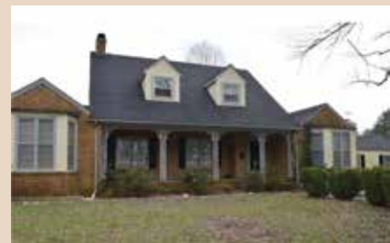
828939 313 GRACE ST., MT. AIRY - Priced well below appraisal, this 4 BR, 2 BA home features lg. living & dining area w/hardwood floors, eat-in kitchen w/ stove, refrigerator & dishwasher remaining, enclosed porch on the back & covered porch in the front. Single attached garage..... $169,900
