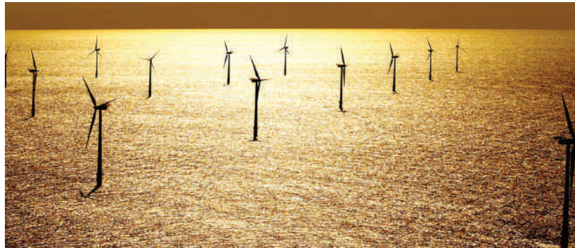
▲ Dong Energy's Horns Rev 2 offshore wind farm (picture courtesy of Elsam A/S)
