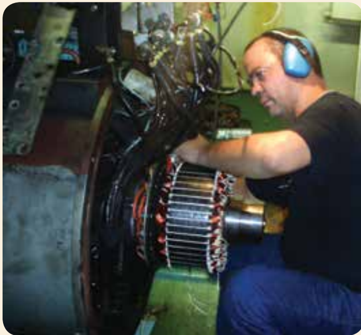
Johnny Canada, technical service manager, Vert Energy, is rewinding an exciter stator, below deck on a vessel in situ, while the vessel is fully operational.
