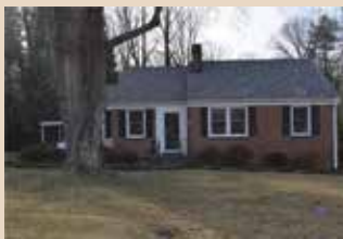
862090 205 FAIRVIEW AVE., MT. AIRY - This dollhouse features 3 BR's, 1 BA w/ shower, kitchen w/appliances remaining & granite counters w/breakfast nook, small sunroom/office, HP/CA (2013) w/ oil piggyback, new roof (2017) & many updates. Small fenced-in back yard, plus bsmt. w/workshop area, insulated windows, walk-in shower & gas logs in fp (not hooked up)..... $139,000
