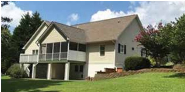
1045 Fox Hills Road, Pinnacle: Quiet country setting w/ 3 or 4 BR & 3.5 BA with so many unique features, custom work & organizational details that it takes hours to identify them all. Must see all the kitchen details, breakfast nook, hall office organizer, Large master suite w/ gas logs, jetted tub, separate shower, custom closets & private office. Maintenance free & beautifully landscaped. Sellers added a screened porch Nutone built-in sound system, private deck 7 garage/workshop, full basement has lifetime warranty against leaks. (MLS# 846792)..... $234,000 Call Bryant at 336-325-7102
