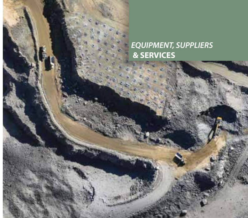
Aerial view from a camera mounted to a small UAV clearly showing the hole positions in the drill pattern.
