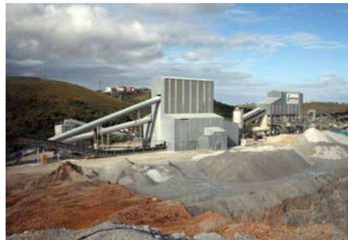
A well-oiled machine: Photograph shows the plant which consists of the primary, and the secondary and tertiary.
