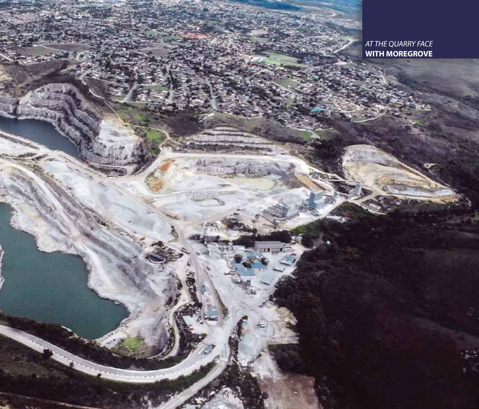
Aerial photograph of the Moregrove operation in Port Elizabeth. Note its close proximity to its neighbours (Courtesy Lafarge Moregrove).
