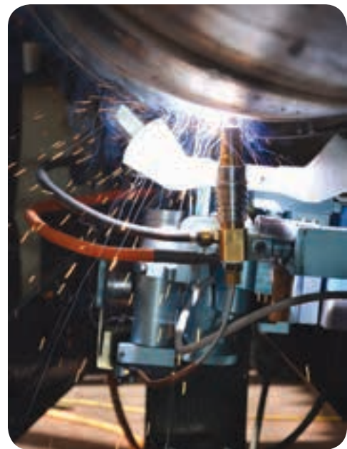
The Gridweld buggy going past the overhead position.
