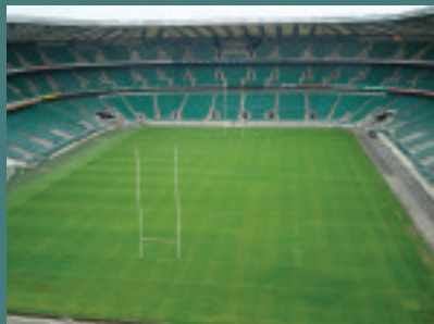
▲ Saint-Gobain Pipelines' rainwater systems were recently specified for the redevelopment of Twickenham Stadium
