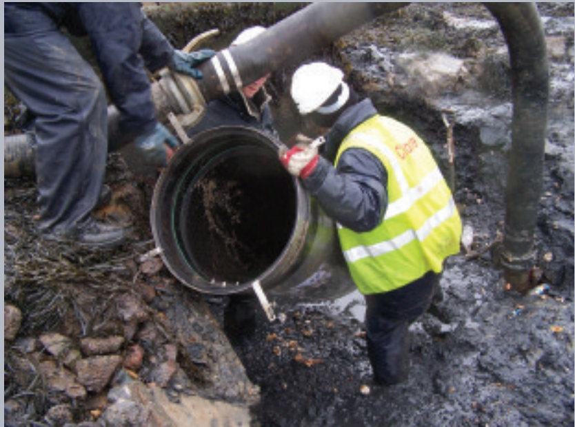
▲ The WaStop check valve from Wapro can be installed quickly and easily
