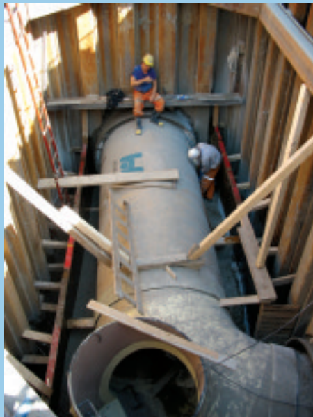
▲ Trenchless installation was used, due to the limited space on-site
