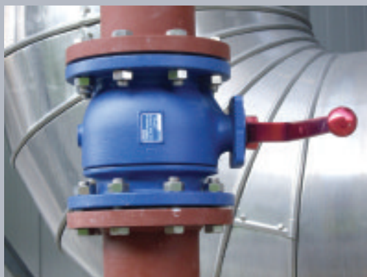
▲ ETEC's ceramic/steel ball valve in operation in a power station
