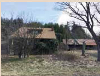
59384 7229 FANCY GAP HWY., FANCY GAP, VA - Formerly operated as The Olde Homestead Mall with a deli, retail area, historic post office & storage space fronting Hwy. 52 in the heart of Fancy Gap. Convenient to I-77 & The Blue Ridge Pkwy..... $150,000
