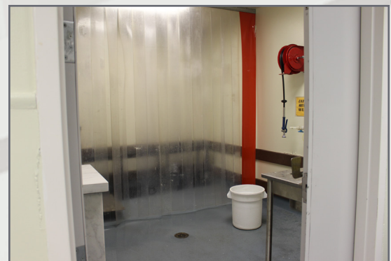
Pictured: Equipment wash room
