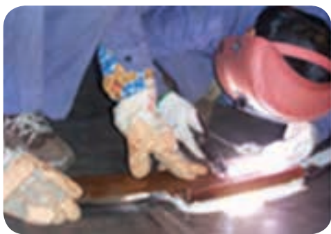
Figure 6. GTAW and plasma welding being applied to the sleeve joint.
