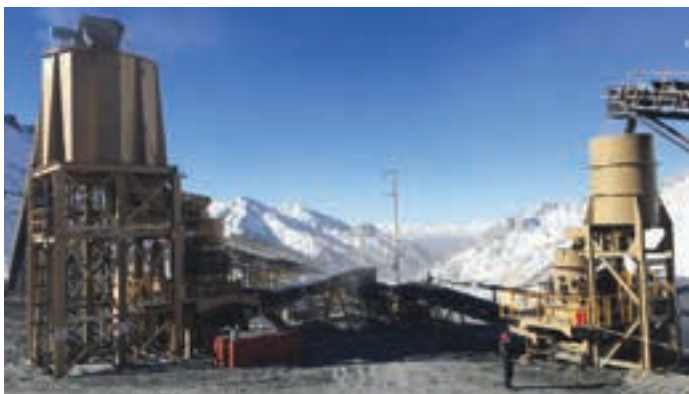
Osborn modular plant operating in testing conditions at the Dundee iron ore processing plant in China's Xinjiang Province.
