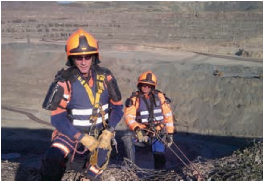
Rope climbers in full safety gear working on the Orapa contract.
