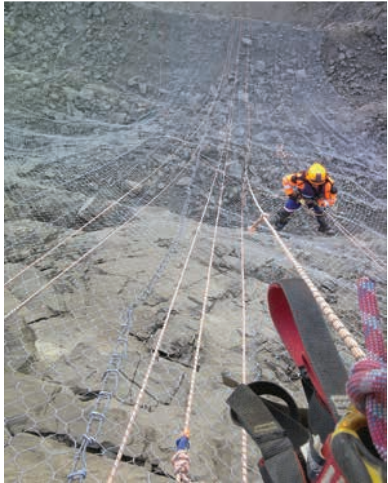
Inspecting the integrity of the drapery mesh system.
