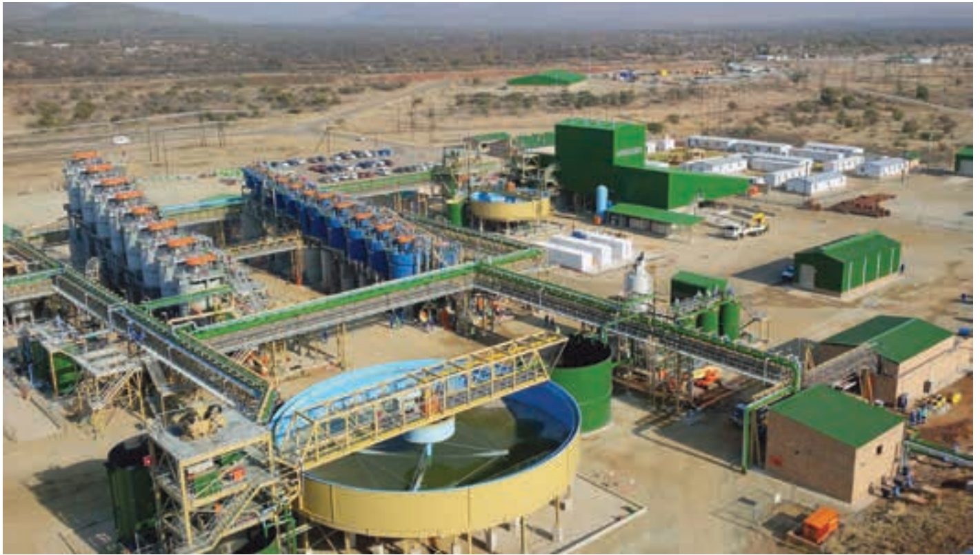
A recent view of the WBJV Project 1 processing facility showing the flotation circuit, concentrator and filter press (photo: PTM).
