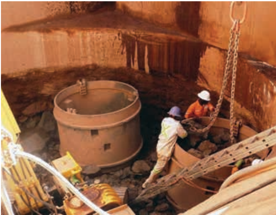
Shaft-sinking activities underway in the Platreef's Shaft 1 (photo: Ivanhoe Mines).
