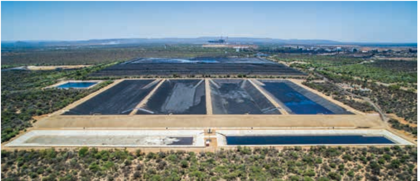
The R385 million cyclic-operated coal slimes ponds facility at Grootegeluk.
