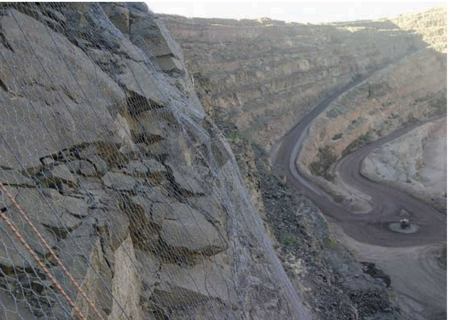
Rockfall protection at Debswana's Orapa diamond mine. Note the proximity of the haul road.
