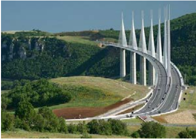
Millau Viaduct, France
