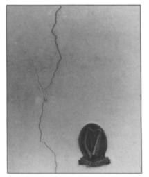
Drogheda Courthouse, Co. Louth – a closeup of the cracks in the wall at the courtroom.
