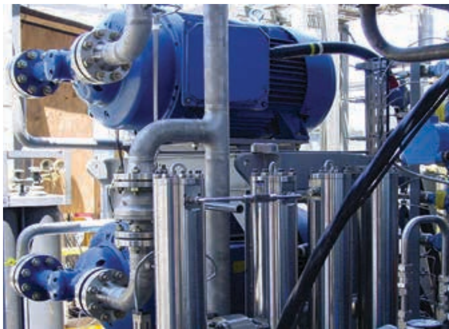
Left: A high head, low flow direct-coupled Pitot-tube Roto-jet pump. Right: The Weir Minerals team installing a Floway VTP pump.
