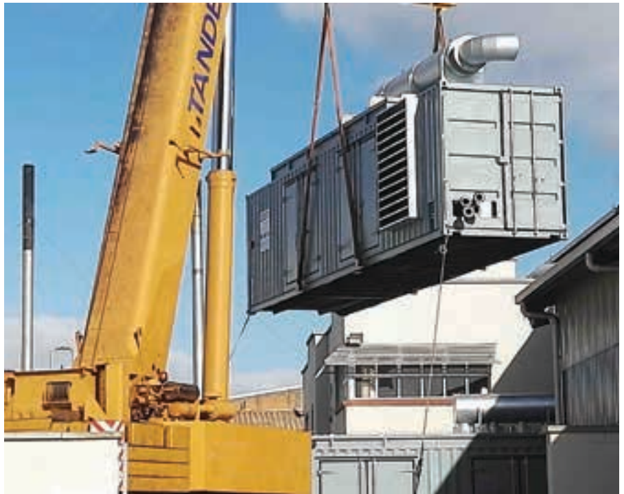
The complete 35 t packaged diesel generator set being lifted for loading onto transport vehicle.
