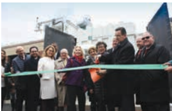
A 2.2 MW fuel cell came online at a regional high school in Connecticut in January 2017. The fuel cell is linked to a microgrid and will power the school during a prolonged power outage. Waste heat from the fuel cell will also be used to heat the high school.
