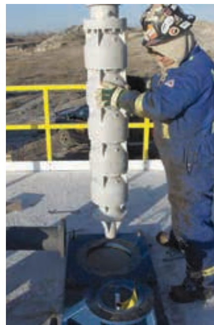
Left: A high head, low flow direct-coupled Pitot-tube Roto-jet pump. Right: The Weir Minerals team installing a Floway VTP pump.
